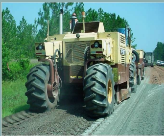
Recycling an asphalt road with cement
