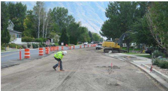
Fig. 1. Marking the perimeter of a treatment area.
