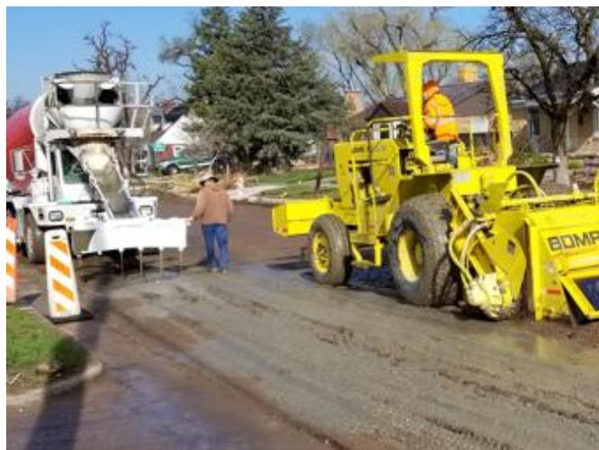
Fig. 5. Simultaneous cement slurry application and reclamation operation in adjacent treatment areas.
