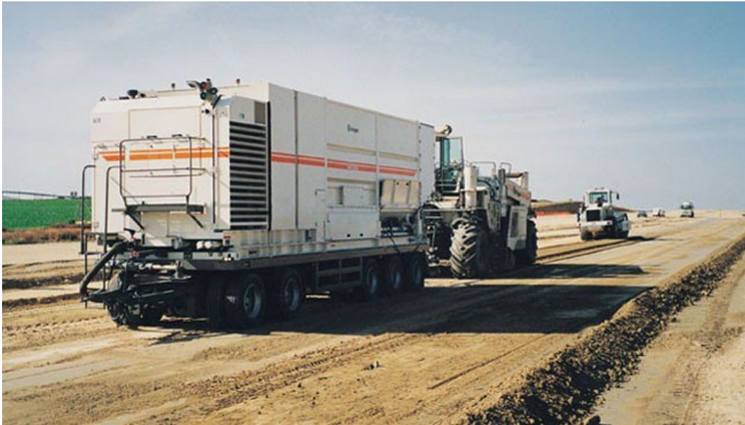
Slurry Train – Slurry injected into mixing chamber
