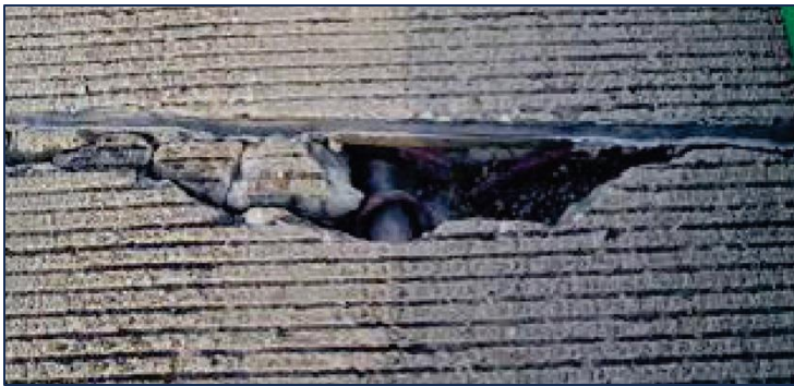
Joint Spalling
