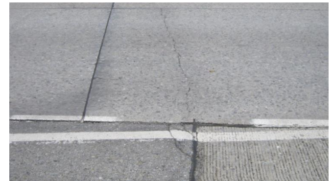
Crack Propagation
