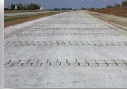
Jointed Plain Concrete Pavement (JPCP) OR (CPCD)
