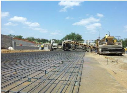
Continuously Reinforced Concrete Pavement (CRCP)
