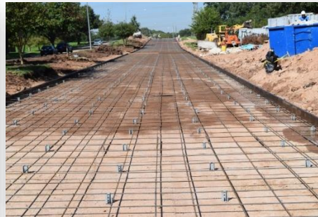
Jointed Reinforced Concrete Pavement (JRCP)
