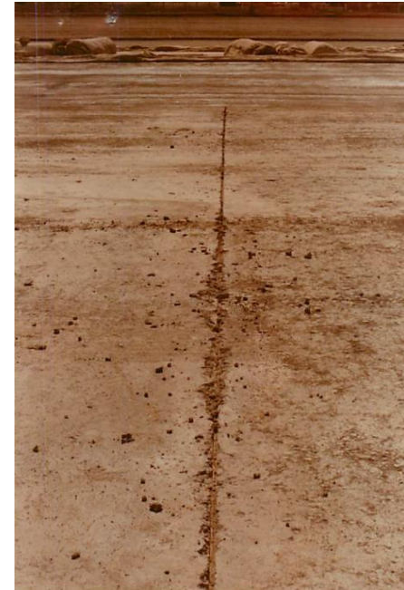
Typical Sawed Joint – Note surface Spalling
