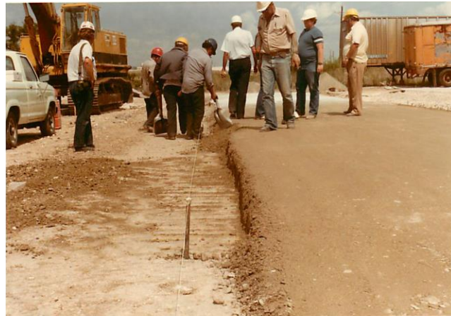
Cold Joint Preparation
