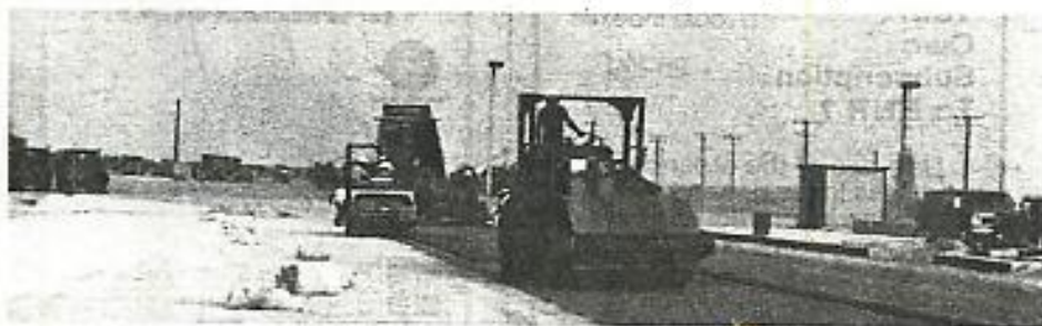
Army parking lot constructed using roller-compacted concrete for added strength.
