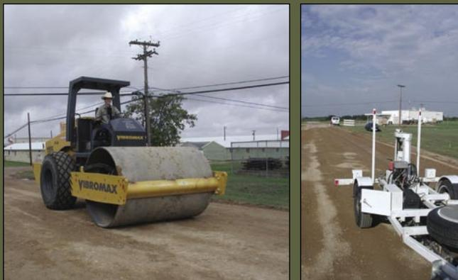
Microcracking in progress with the vibratory roller. TxDOT's FWD can serve as the control mechanism to determine when to stop rolling by measuring the reduction in average base modulus.
