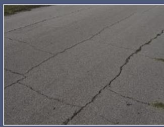
*Block cracking typical of CTB.*
